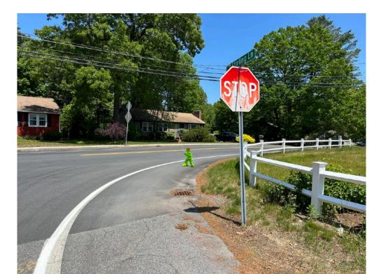
This \$30 piece of plastic has done an incredible job slowing down cars which would previously take tight turns here at high speeds, acting as a de-facto slip-lane despite the stop sign.
