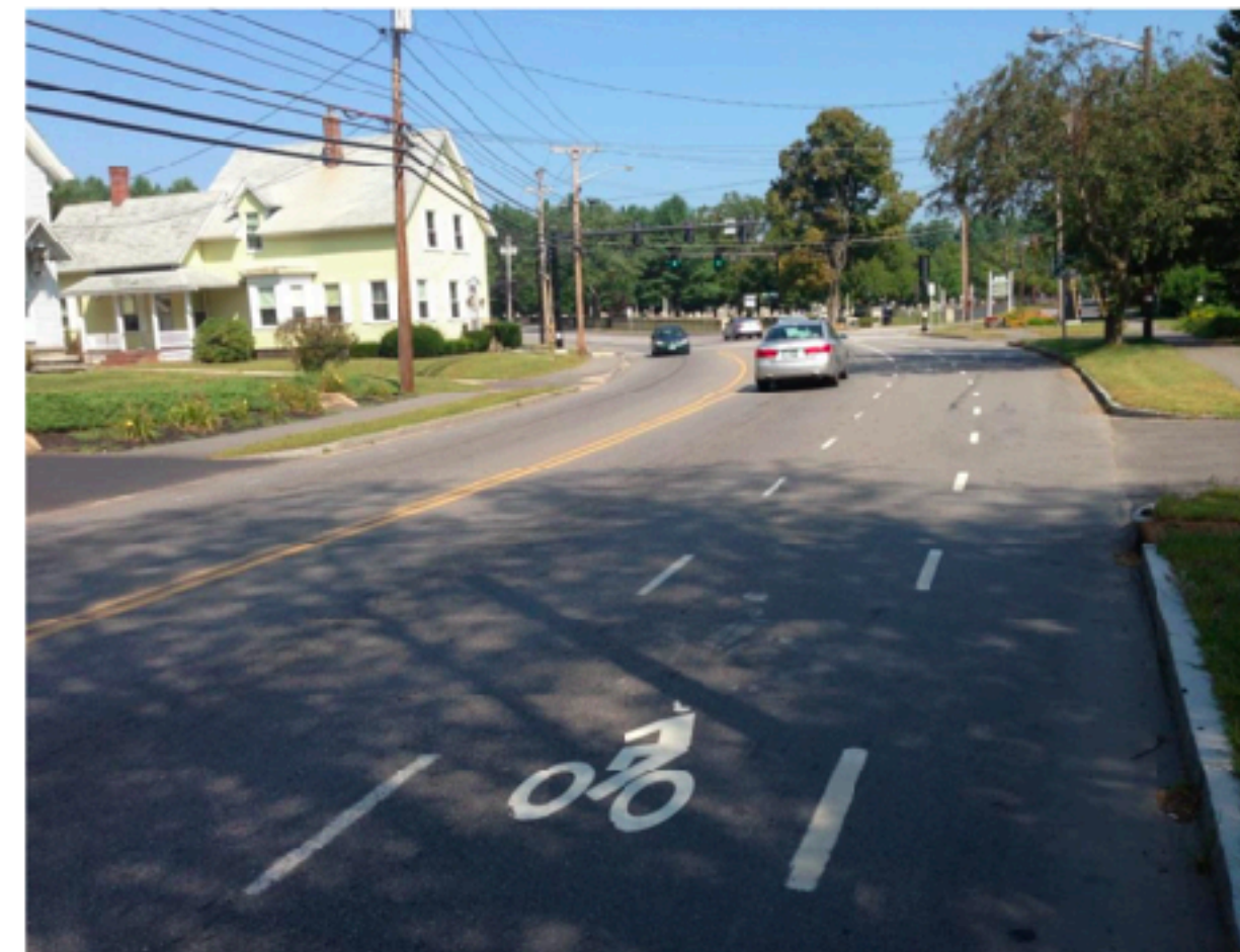
One of Concord's most visible examples of its new 'Complete Streets' policy is the US Route 3 Improvements Project which will include fully-compliant bike lanes from downtown Concord to Penacook Village
