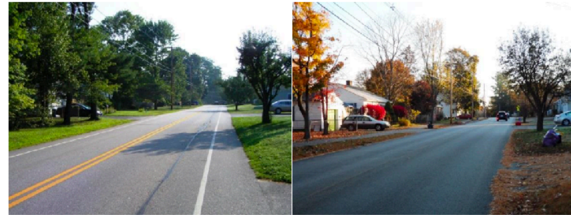
Left: Lane narrowing and shoulders prior to sidewalk construction. Right: After sidewalk construction.
